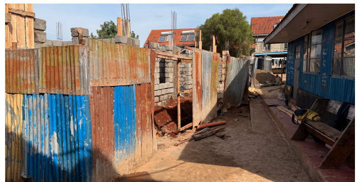
Construction work at the Mothers' Mercy Home
