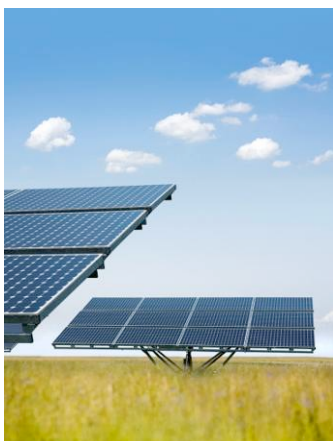
A Solar Power
